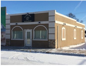
Front of Building
