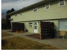
3 apartments lower level
