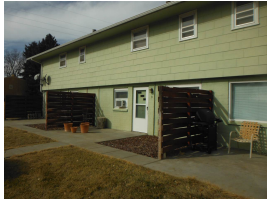
3 apartments lower level
