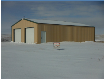
30' x 48' Cleary Building
